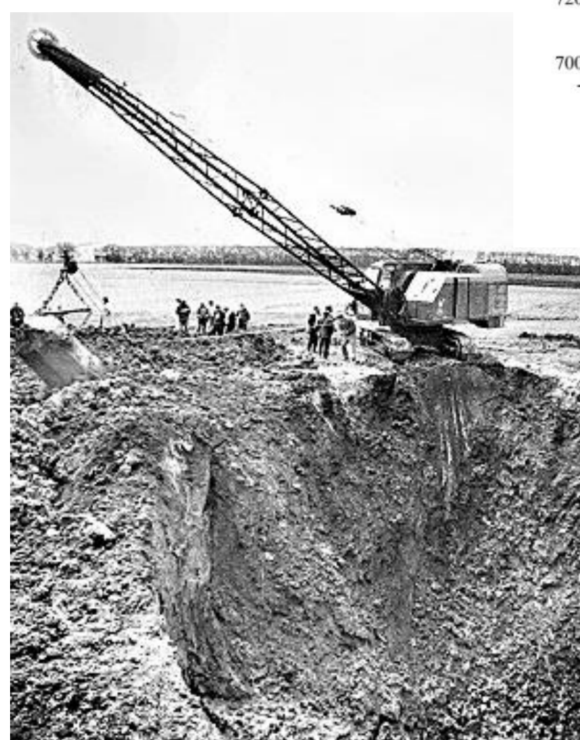
The first stage of the search and excavation using an excavator
