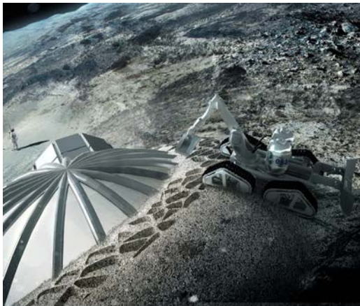
Fig 1: a possible step towards the MoonVillage using robotic with 3D printing to consolidate inflatable domes against radiation and meteorites before the arrival of astronauts
