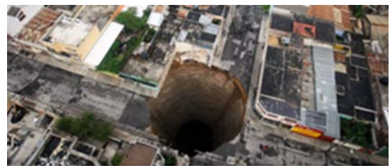
Figure 3. 2010 Guatemala sinkhole (National Geographic)
